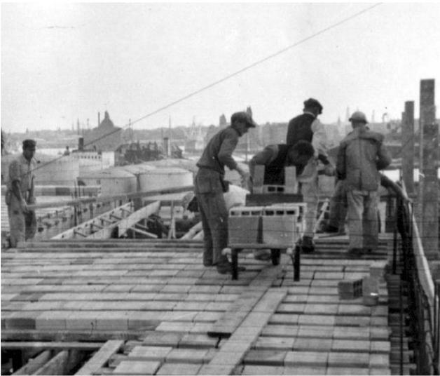
Figure 6. Construction of the first prestressed steel-brick roof, Pakhus 47 (Warehouse 47) in Copenhagen, 1948 (Copenhagen Museum).
