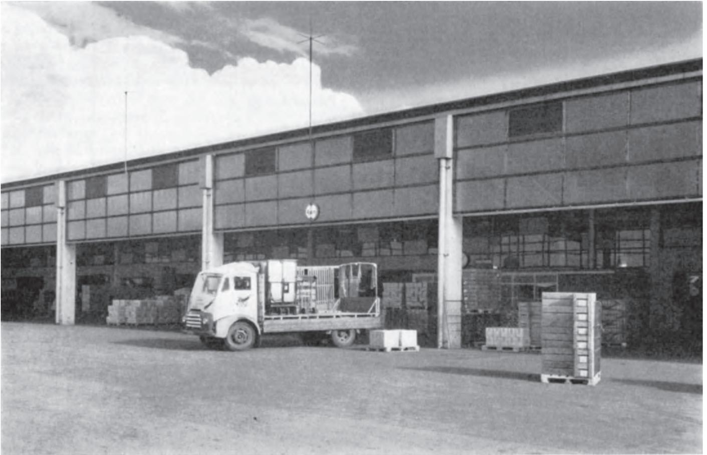
*Even the newly built warehouse for the country's largest grocery company, FDB, did not in the 1960's have access ramps. Trucks performed all-weather transport to deliver goods.*
