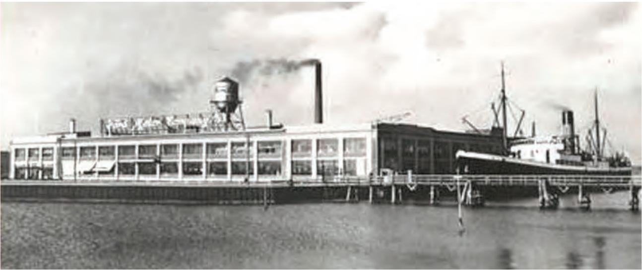
*Ford's assembly plant in 1924 was built from reinforced concrete. It was not until the construction of pre-cast concrete that building large, pillar-free factories was possible.*
