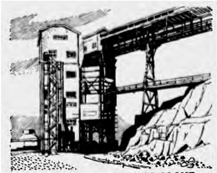
*Figure 4. The ice-making plant for concrete casting at Warragamba Dam. Sydney Morning Herald 13 October 1957, p. 8.*
