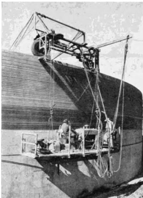
Figure 8. Pre-stressing of a circular concrete tank by the Preload system. *Building, Lighting and Engineering* 24 April 1954, p. 55.
