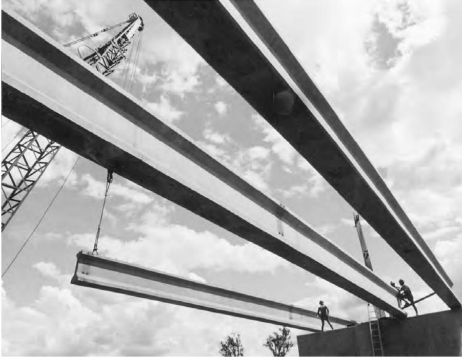
*Figure 1. Pre-stressed concrete beams changed the construction work, as here at O'Shea's Crossing Bridge, John Holland Constructions 1977. Photo: Wolfgang Sievers, National Library of Australia, nla.obj-143341980.*
