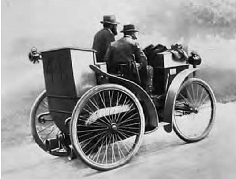
*In 1895 the Michelin brothers presented the first pneumatic tire for cars. Their Eclair racer was equipped with the new tire.*
