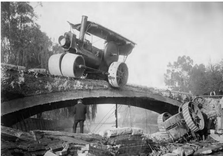
*Fig. 10. The First King's Bridge, Bendigo, Australia did not pass the test in 1901 when two steam rollers tested the construction. Half of the enforced concrete bridge collapsed.*
