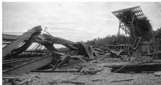
Fig. 5 and 6. The Quebec Bridge should be the longest bridge in the world, but almost finished in 1907 the bridge collapsed and 75 workers were killed.
