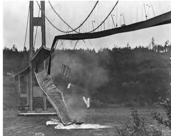
*Fig. 11. The probably most famous bridge accident is the collapse of the Tacoma Narrows Bridge, Washington. Under a storm it began to move vertically and collapsed few months after it opened to traffic in 1940.*
