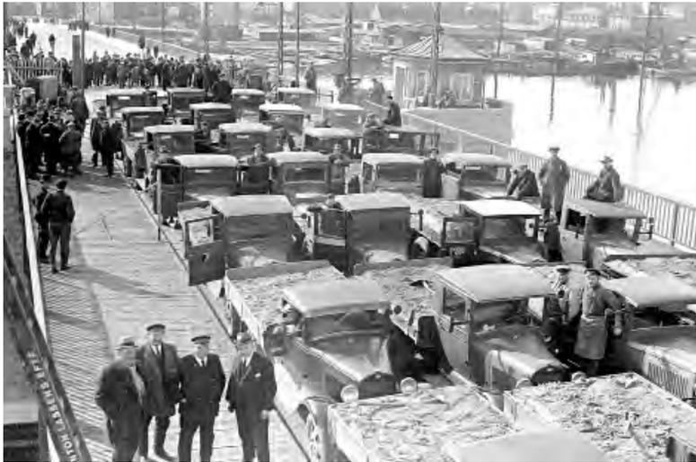
*Fig 9. The new built Limsfordsbroen, Aalborg, Denmark, was tested by 48 heavy loaded trucks in 1933.*
