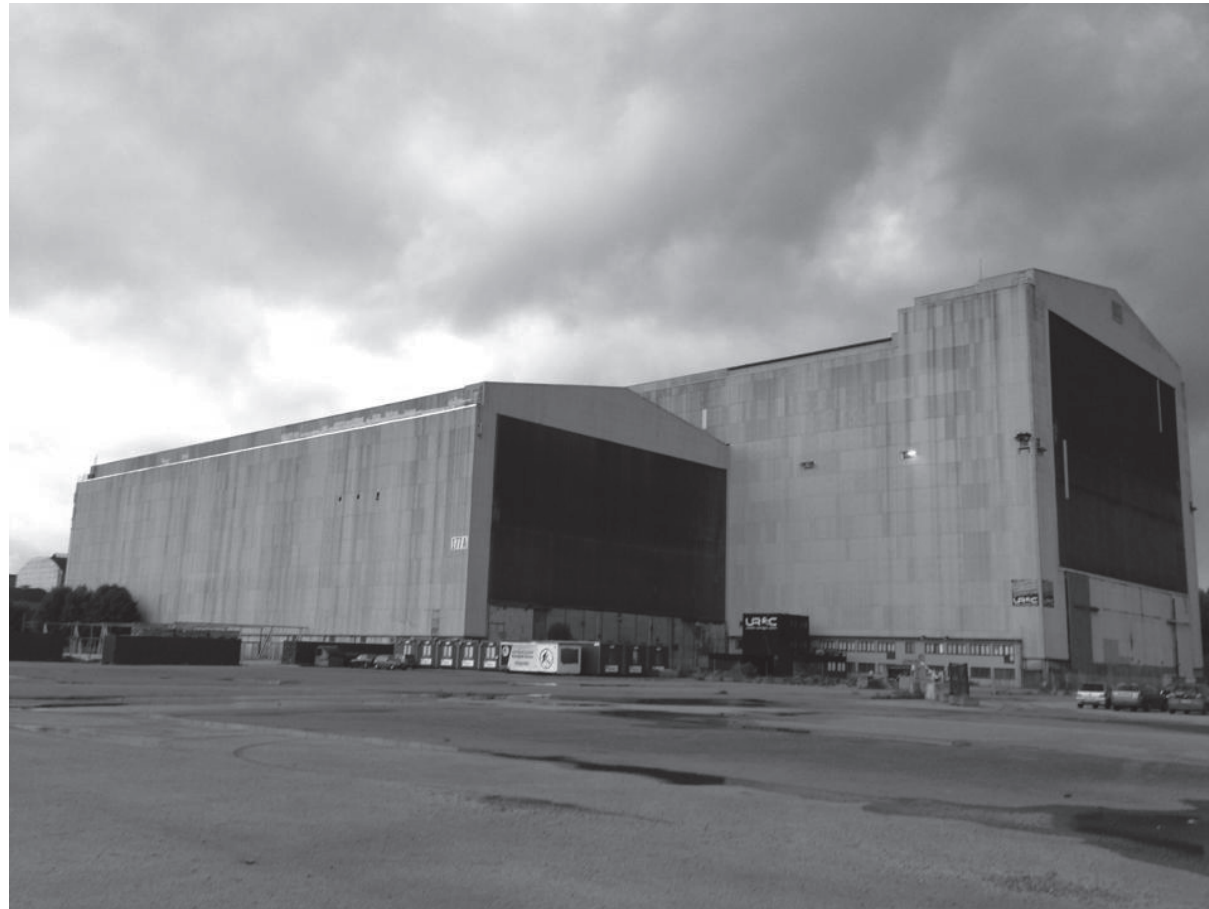
Fig. 2. The shipbuilding halls, built in the early 1960s for the now-defunct B&W shipyard in Copenhagen, are among the 25 buildings nominated by the Ministry of Culture for being worthy complexes for Danish industrial culture. Photo: © Politikeren, Wikipedia, 2013.
